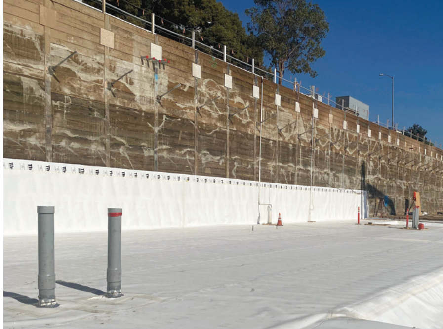
First course of blindside waterproofing applied against soldier pile lagging.
