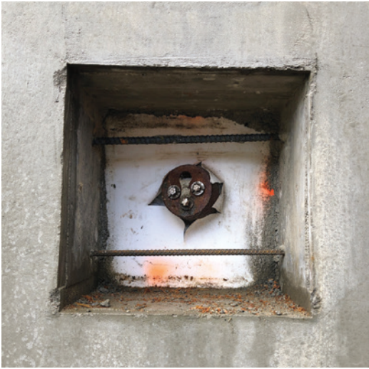
A detensioned tie-back ready for application of blindside waterproofing patch.
