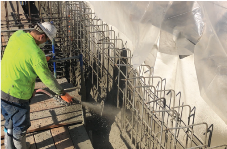
Shotcrete application against installed blindside waterproofing membrane.
