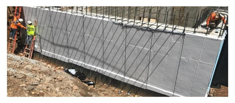
Self-adhesive, waterproofing membrane and vapor retarder Strong, pliable rubberized asphalt membrane with HDPE backing
