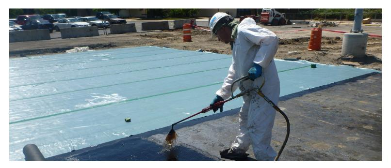
Hot fluid-applied polymer rubber gel composite membrane system Self-healing, non-curing, versatile, fast application
