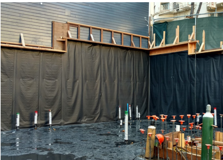
NovaTak fuses to concrete through an ionic chemical reaction.
