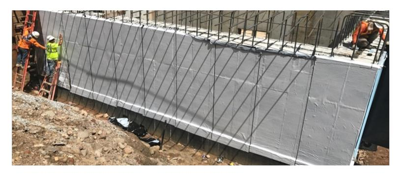
Self-adhesive, waterproofing membrane and vapor retarder Strong, pliable rubberized asphalt membrane with HDPE backing
